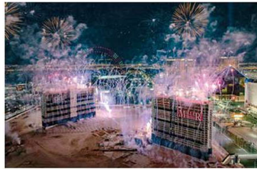
Photo credit GGG Demolition
